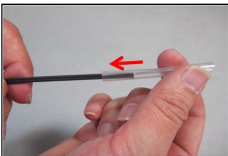
3: Insert a protection sleeve over the cable.
